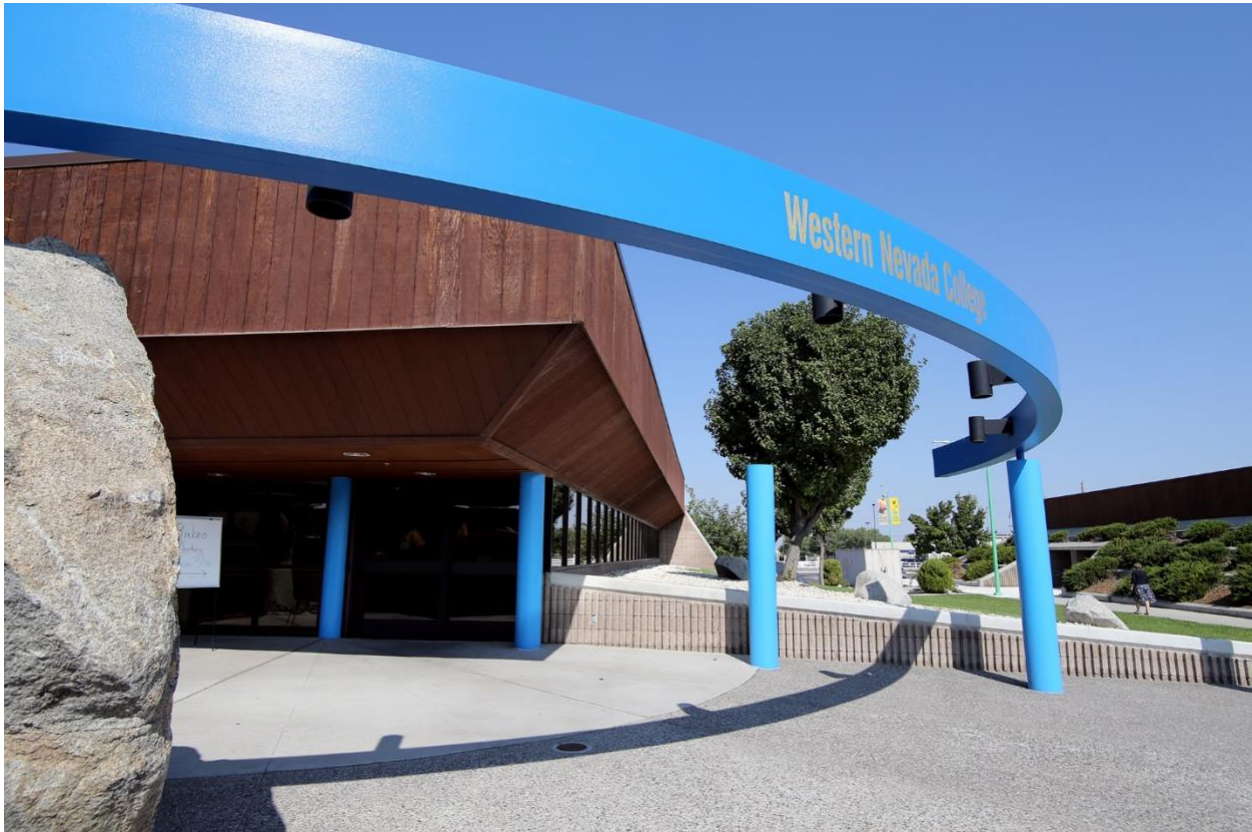
Fallon Campus – Getto Hall
